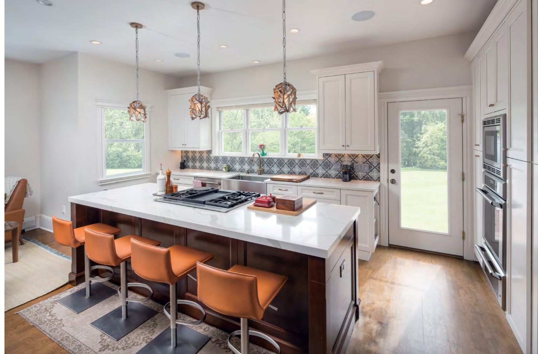
▲ The cabinet to the left of the exterior door was custom built with a false decorative panel on the front and an open side on the end for storage.
